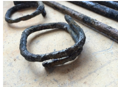
Figure 3 Figure showing Corroded Reinforcement
